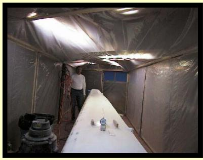
I wasn't sure what to tackle next, but finally decided to spray the leading edge with a coat of Prestec to restore the leading edge sharpness ... and just to build material to prevent breaking through on the final sanding. A couple of commercial refinishers stressed the need to have additional leading edge material on the wing. I basically just sprayed the LE and extended the pattern 6" on top and 3" on the bottom. I then turned
